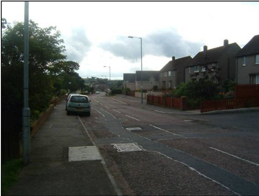
Photograph 3: Footways on Strathaven Road west of Teiglum Road junction
